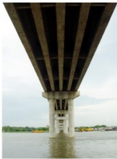
P.C. Girder Bridge
