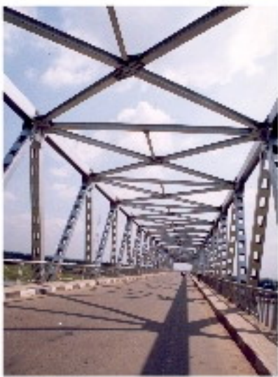
Steel Truss Bridge
