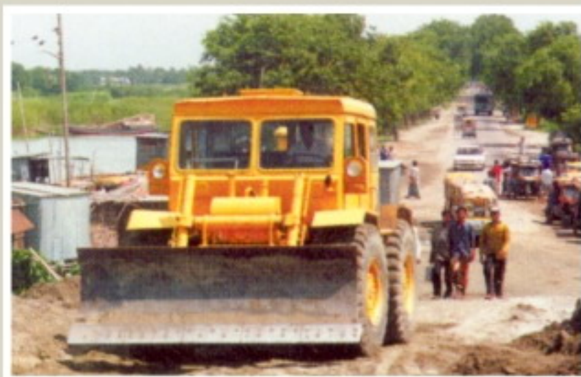
Heavy Earth Moving Work
