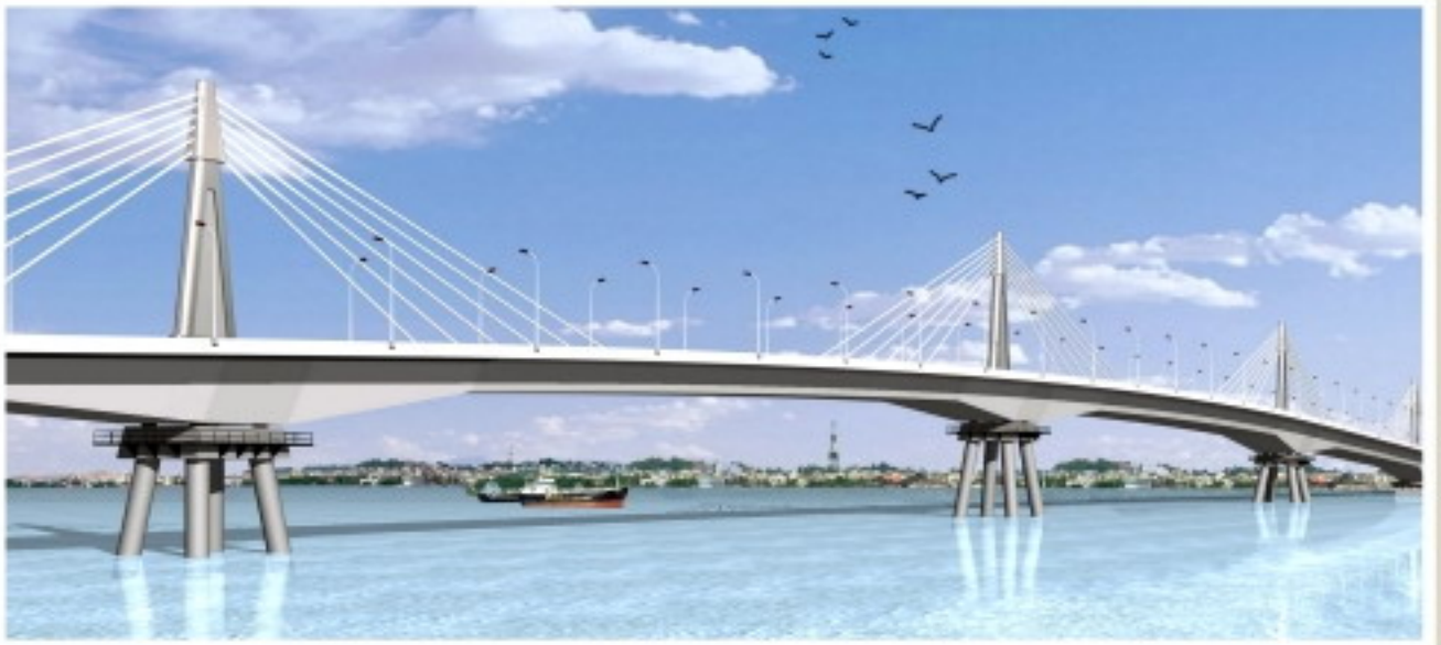
Extra dozed PC Box Girder Bridge
