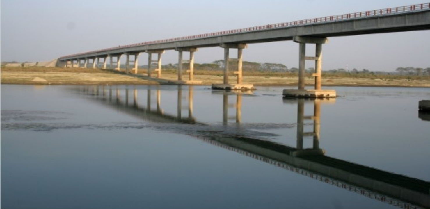
Pre-stressed Concrete Girder Bridge
